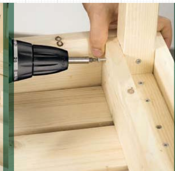
4. Fit the reinforcement panels
