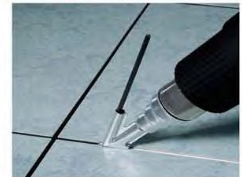
Welding Plastic Tiles
