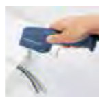
Cutting out small cable channels
