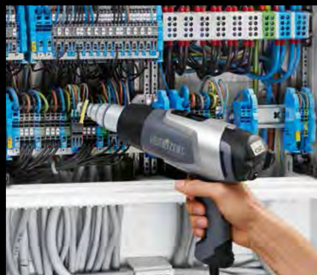
Shrinking cable sleeves in distribution cabinet
