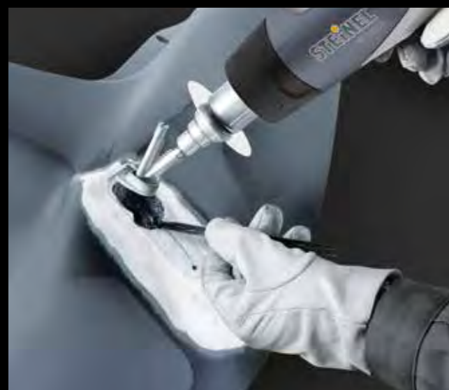
Repairing crack in bumpers.
