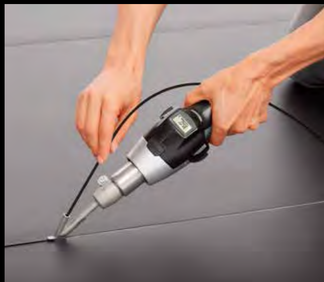
Welding linoleum floors.
