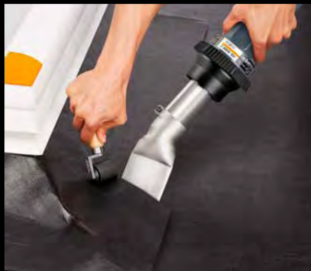
Overlap welding on a light dome.
