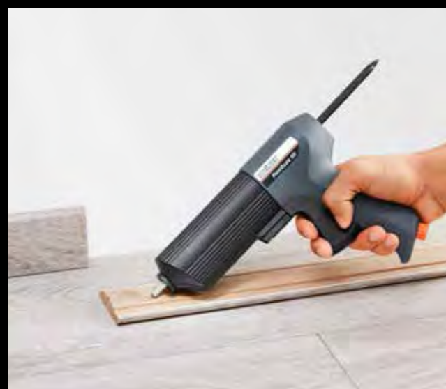
Gluing on skirting boards for permanent attachment.
