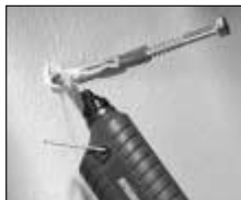
Securing loose wall plugs.
