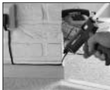
Laying telephone cable.
