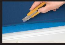
If the tape pulls paint up with it, try lightly scoring the edge of the tape with a razor blade before continuing to remove tape.
