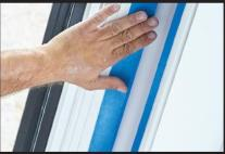
Press down as you go, using your fingers to lay tape into surface depressions.
