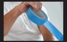
Tear off about 2 to 3 feet of tape at a time, laying each new piece of tape over the end of the previous piece.
