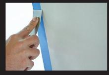
Secure tape by pressing the edge down with a putty knife or 5-in-1 tool. For textured surfaces, seal the edge of the tape with the existing base paint color of the wall.
