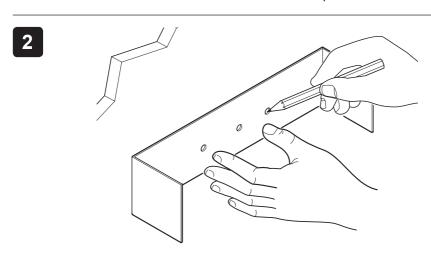
Mark the positions of the fixing holes on the wall.
