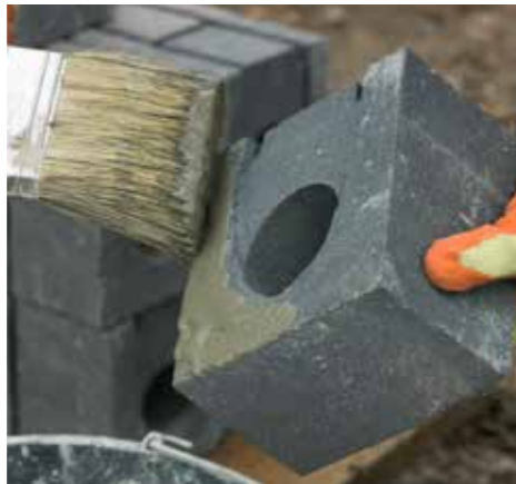
3. Before installing the Drainar units, apply a 5mm bead of M-Flex or paste M-Fix compound from the top of the aperture.
