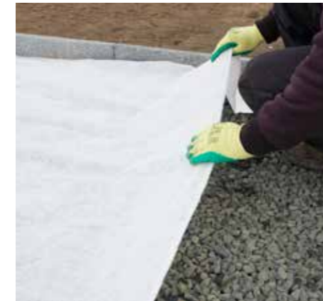
3. Place Geo-textile on top of the clean crushed stone.
