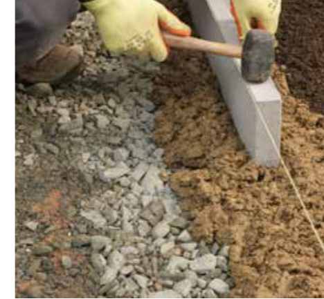
1. You must install your choice of edge restraint on a concrete footing around the perimeter of the pathway
