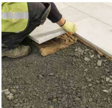
5. Install the paving using the laying pattern.
