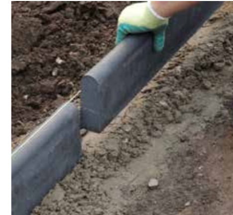
1. Install your choice of edge restraint on a concrete footing around the perimeter of the patio.
