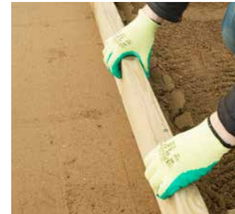
3. Compact first layer of sand and screed out a 30-40mm sharp sand bed
