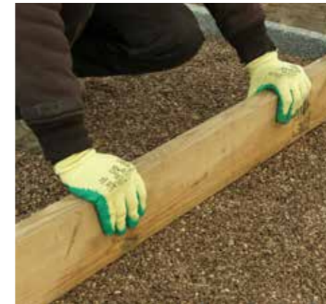
3. Prepare your laying course using 50mm of 6mm clean crushed stone. Only light compaction required.
