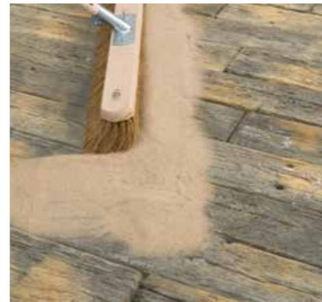
6. Fill joints with kiln dried sand, using a stiff broom.
