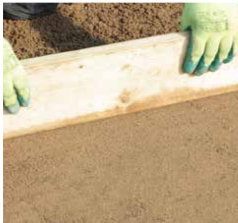
3. Compact first layer of sand and screed out a 30-40mm sharp sand bed.
