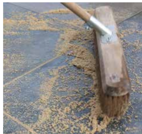
6. Brush in Stonemarket Narrow Jointing Compound following the instructions on the tub, using plenty of water.
