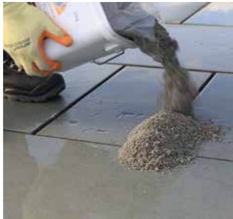
3. The Fast Point material is poured onto the wet paving
