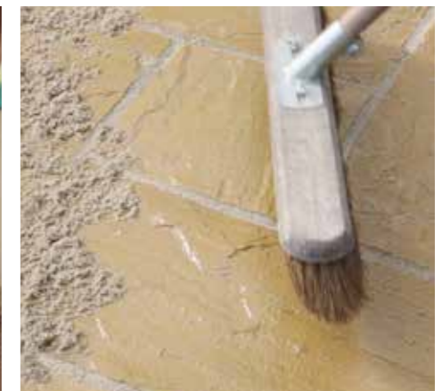
6. Brush in Stonemarket FastPoint following the instructions on the tub, using plenty of water.
