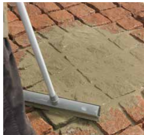
6. Joint using Instamac Flow Point following the instructions on the pack.
