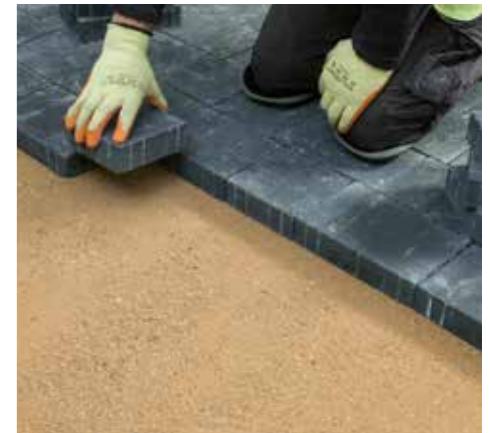
4. Install your choice of paviers using the laying pattern, spacers will be provided if the products don't feature nibs.
