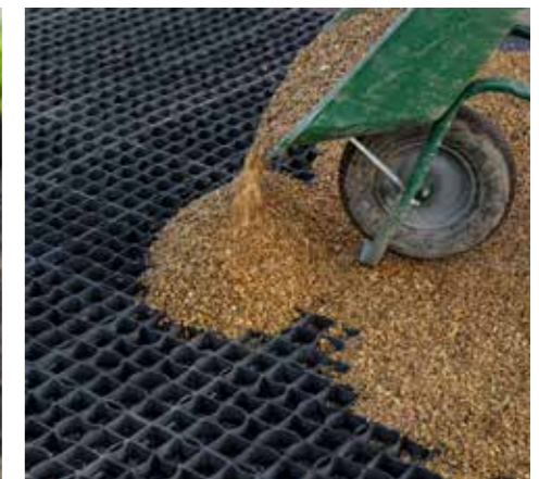
6. Fill the Drivegrid with the supplied 6-10mm aggregate. Coverage allows for a 10mm layer above the cell height.
