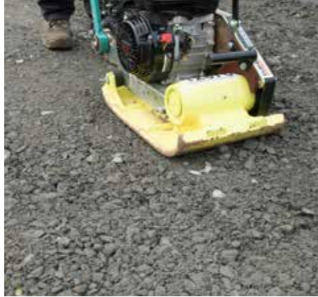
1. Prepare the ground as normal with compacted hardcore, achieving the correct falls for drainage.
