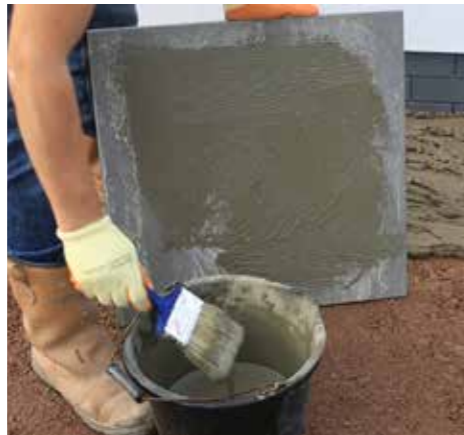
3. Paste to the rear of the paving a slurry backing prior to laying.
