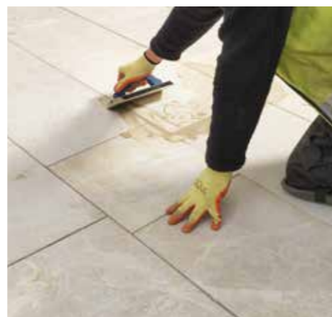
6. Joint using a waterproof external grout following the instructions on the tub.
