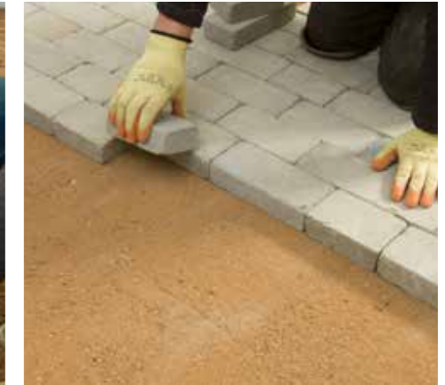
4. Install the setts using 1-2mm spacers, using a laying pattern.
