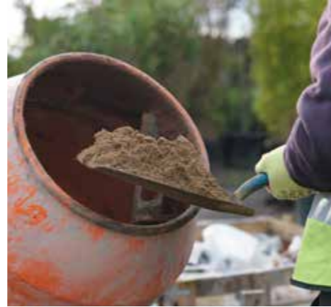
2. Mix a wet mortar mix of 1 part cement to 5 parts building sand.
