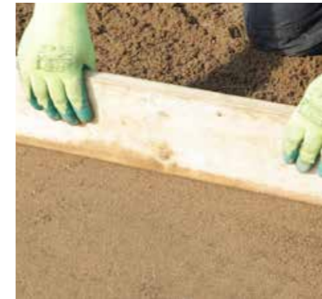
3. Compact first layer of sand and screed out a 30-40mm sharp sand bed.
