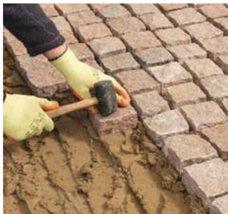
5. Install the paviers using the laying pattern keeping a consistent joint width.
