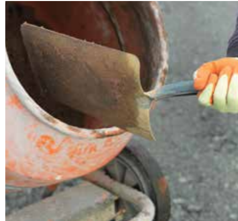
2. Mix a wet mortar mix of 1 part cement to 3 parts building sand.
