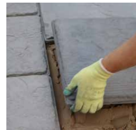
5. Install the paving using the laying pattern.
