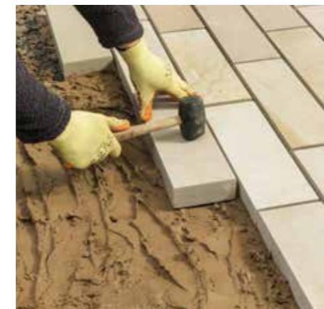
5. Install the paving using the laying pattern.
