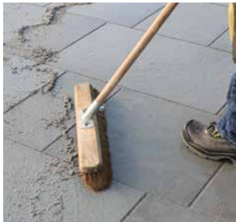
5. Any excess is carefully brushed off. Particles left on the paving may leave a speckled finish.
