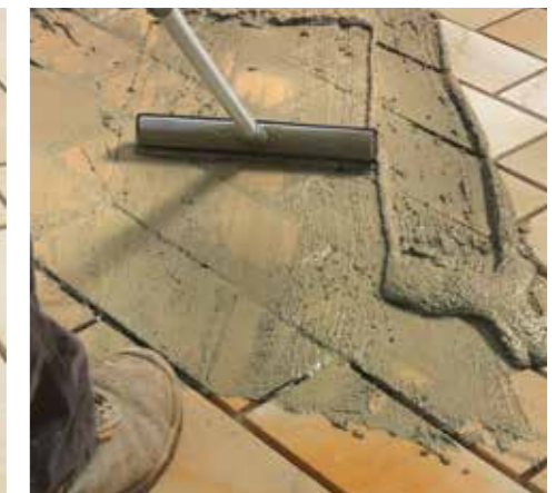
6. Joint using Instamac Flow Point following the instructions on the pack.
