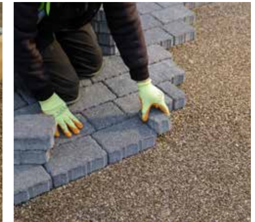
4. Install your choice of paviors using the laying pattern.
