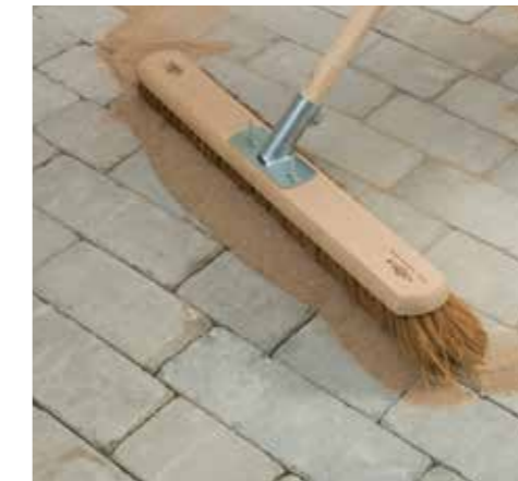
5. Fill joints with kiln dried sand, using a stiff broom.
