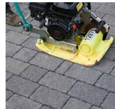
5. Using a plate vibrator compact the blocks.
