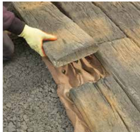
5. Install the paving using the laying pattern.
