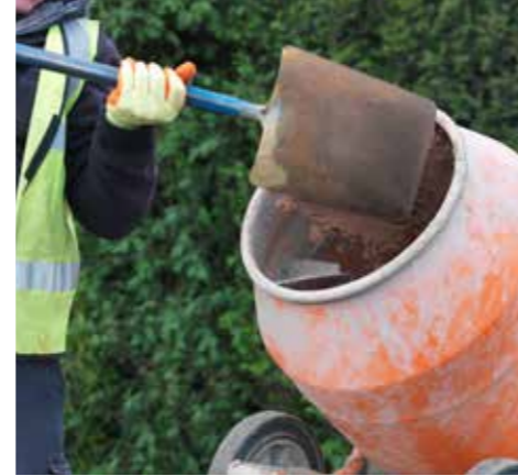
2. Mix a wet mortar mix of 1 part cement to 5 parts building sand.
