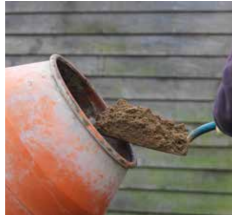
2. Mix a wet mortar mix of 1 part cement to 5 parts building sand.
