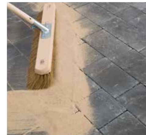
5. Fill joints with kiln dried sand, using a stiff broom.
