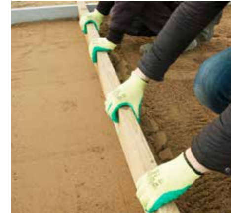
3. Compact first layer of sand and screed out a 30-40mm sharp sand bed.
