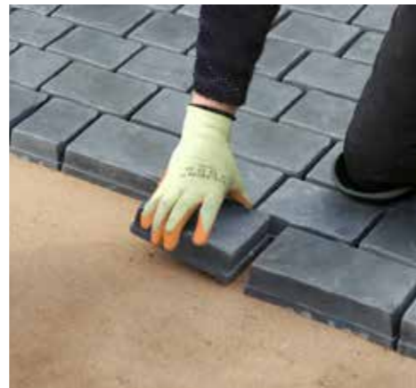
4. Install the engineered Templeton or Millstone Driveway Setts
