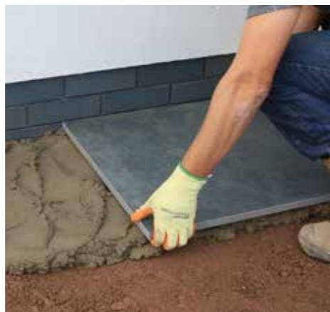
5. Install the paving using the laying pattern.
