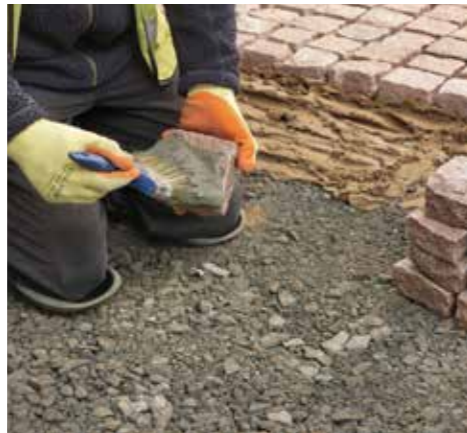
3. Paste to the rear of the paving a slurry backing prior to laying or dip into a pre prepared rhino tub of slurry backing.
