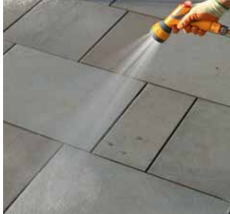
1. The paving is soaked with a hose. Keep wet throughout to avoid temporary staining.
