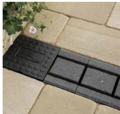
6. Lay the paving flush with the top of the Drainar units. Accessories are available, please ensure you read through the full Drainar installation and maintenance guide.
