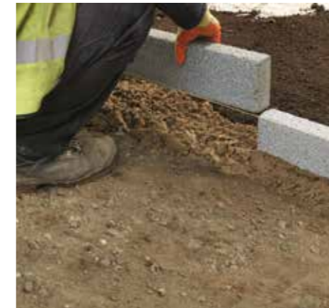
1. Install your choice of edge restraint on a concrete footing around the perimeter of the patio.
