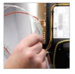
With the self tapping screws partially fitted to the fixing locations in the front casing, carefully offer it onto the back plate assembly ensuring the wires are not trapped. The control knob, in the fully cold position, may have to be slightly adjusted to enable the keyways to align.
