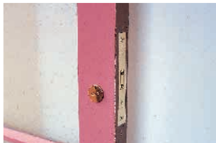
The lock & escutcheon plates fully fitted.
