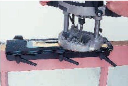
Routing the recess for the faceplate.
