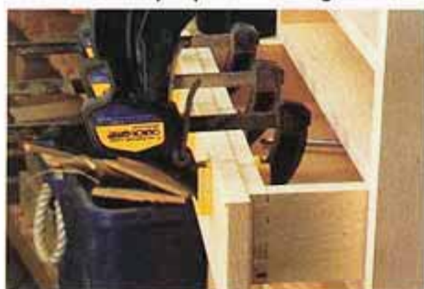
36 Carefully position each drawer front, then clamp in place until the glue sets.
