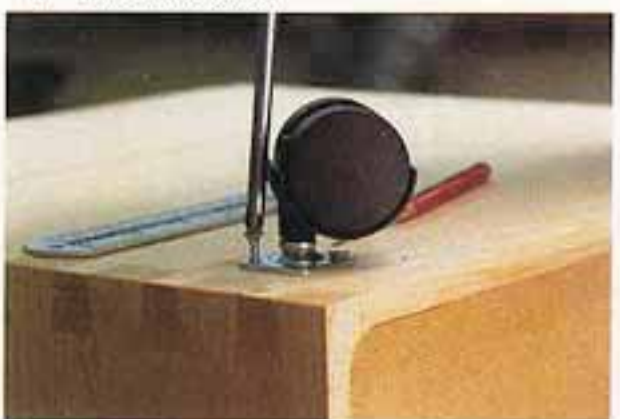
44 Screw the castors onto the base.
