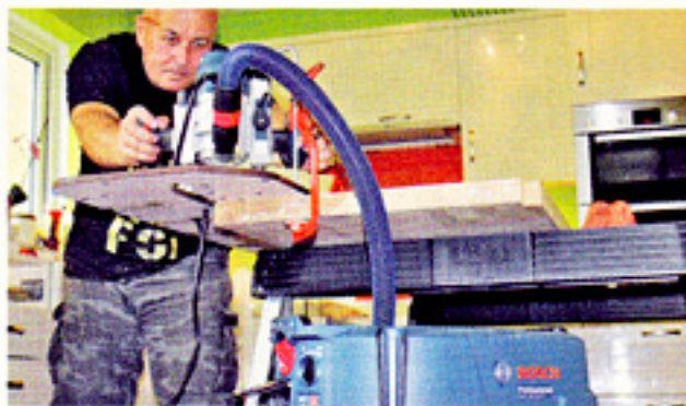
▲ Take a number of passes to ensure a clean cut and make the mating cut on the opposing piece
