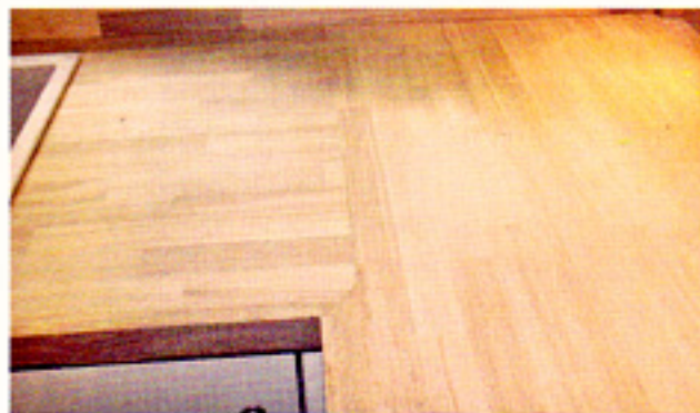
▲ Once bolted up the joint is spot on – as tight as a drum
