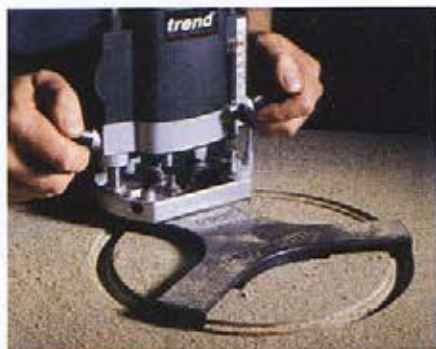
Simply rout a circle to create an access hole
