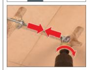
Turn hex bit to tighten Zipbolt and to tighten joint.
