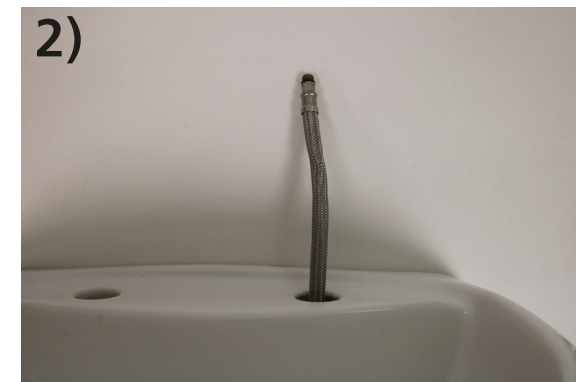
2) Push one of the FlexiTales through the desired tap-hole
