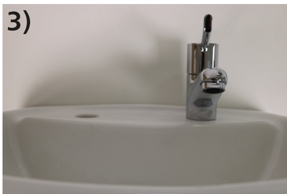
3) Attach FlexiTale to the base of the tap and position the tap in place over the tap-hole
