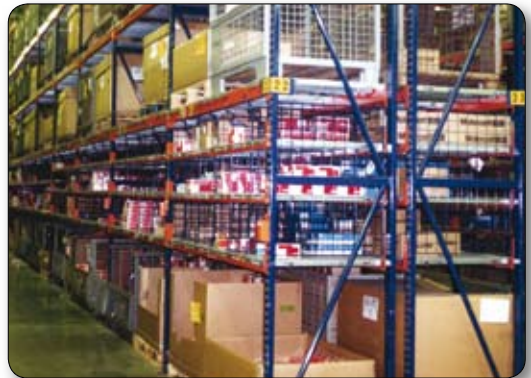
Warehouse racking, Ford, France
