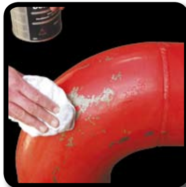
Cleaning and degreasing
