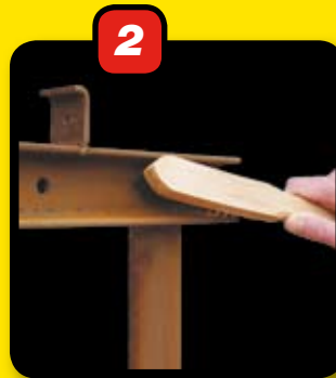
Manually derusting and degreasing
